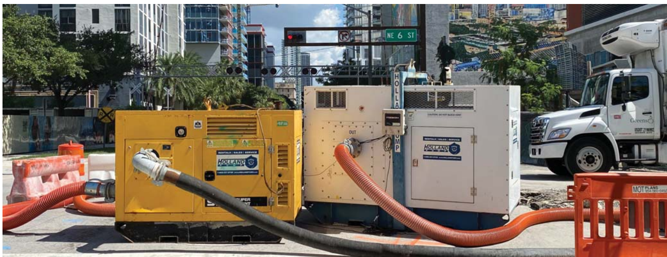
Holland Pump, contracted to dewater the deepest underground parking garage in Miami, uses multiple 4-inch Holland hydraulically driven submersible pumps from a depth of more than 30 feet.
