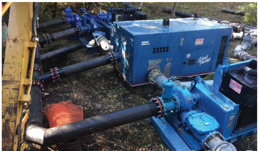
Below: Six-inch suction lift pumps working on a sewer bypass in Jacksonville, Fla., to repair a line.
