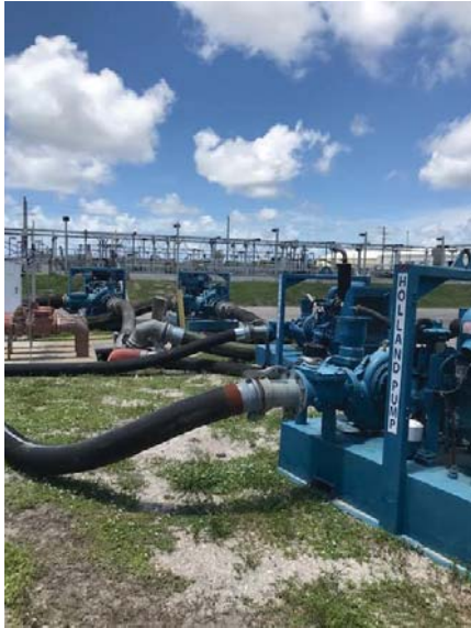
Holland 8-inch and 12-inch suction lift pumps on a bypass at a major lift station in South Florida. The station pushes 7000 GPM at 130 TDH. Photo by Holland Pump
